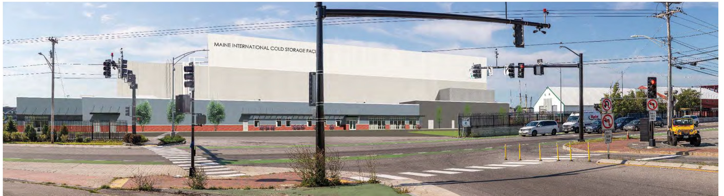
BUILDING VIEW 4: VIEW FROM BEACH STREET (AT COMMERCIAL STREET)
